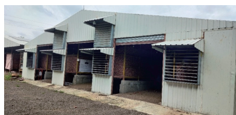
c. Photographic front view of ECOSS with exhaust fan
