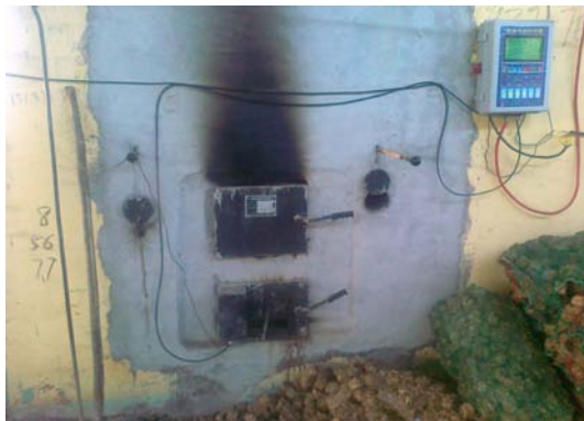
b. Fuel filling process with TSB
