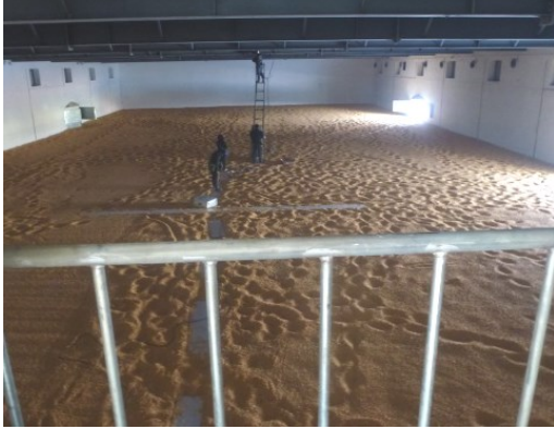
Figure 1 Internal environment of the granary
