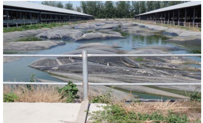
Figure 2 A covered lagoon for storage of the liquid fraction from the slurry separator (on top of the cover, some rainwater has accumulated)
