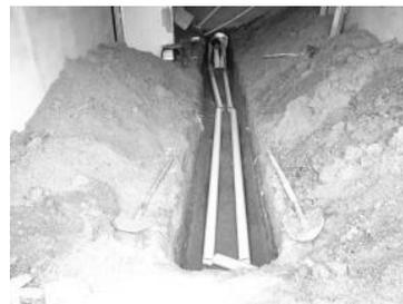
Figure 8 Underground installation of PE pipe
