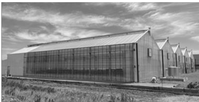
a. A view from the southwest side
