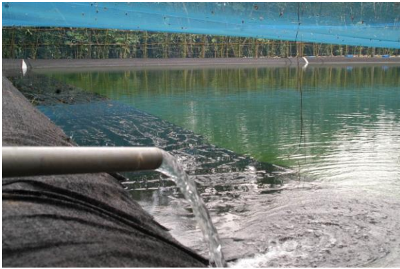
Figure 5 Inflow to the Silpolin lined spring-fed pond
